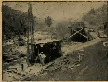
Colusa Natural Oil comes in solution with water. Wells No. 1, 2 and 3, and receiving tanks, into which thousands of gallons of water are pumped for each gallon of oil recovered.
